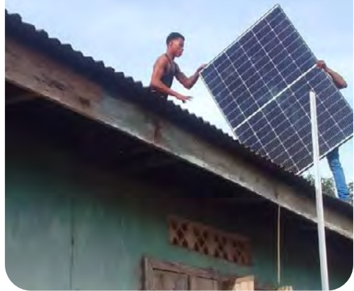
Rooftop solar panels being installed
