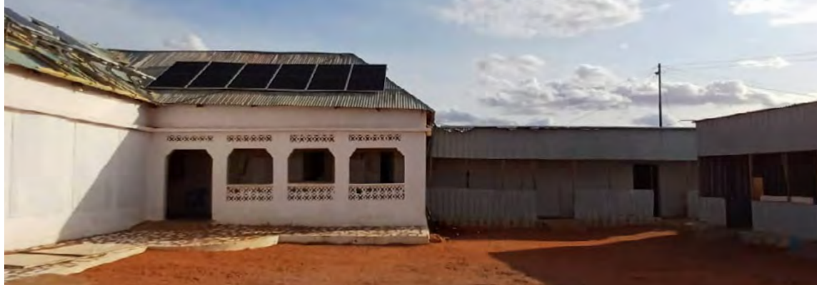
A health facility in Somalia powered using solar PV
