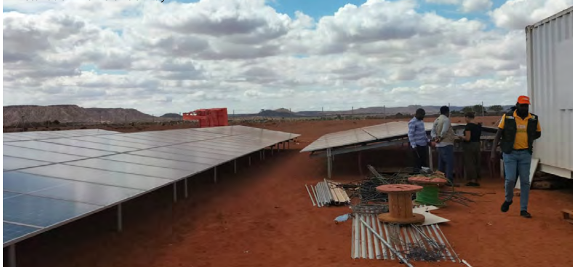
Installation works underway
